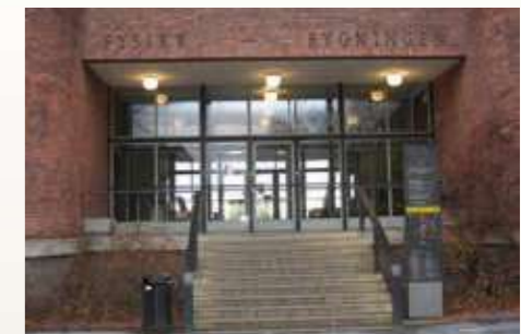
December 2018 University of Oslo Physical restructuring of former labs and construction of new one
